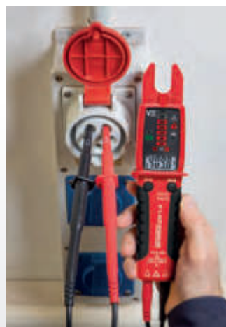
Voltage measurement and phase sequence test
