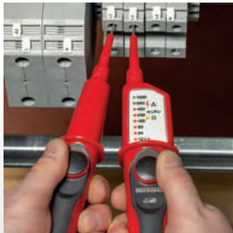
Rotary field test on the output terminals of a UPS
